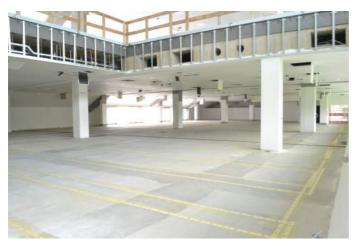
After sanding and priming, the installers then applied Uzin NC 160 self-leveling smoothing compound at a thickness of 2 to 3 mm using a trowel. The compound has low tension, excellent flow characteristics and creates completely level subfloors. The result is a very smooth, highly absorbent surface that reduces the amount of adhesive required for the
